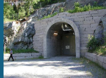
Combined Storage and Repository for Radioactive Waste (KLDRA) Himdalen
