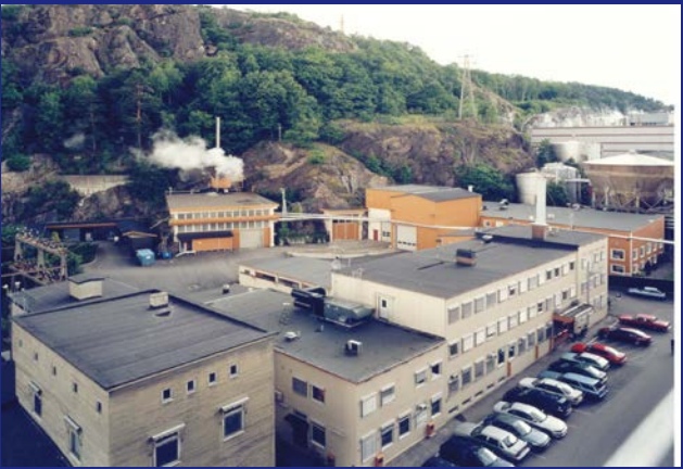
Nuclear Research Facility Halden (HBWR)
