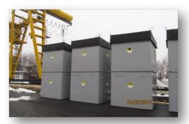
High activity DSRS in their original shieldings are stored in reinforced concrete containers
