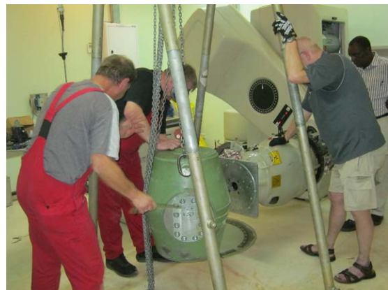
Figure 3: Cobalt 60 source exchange at CDH
