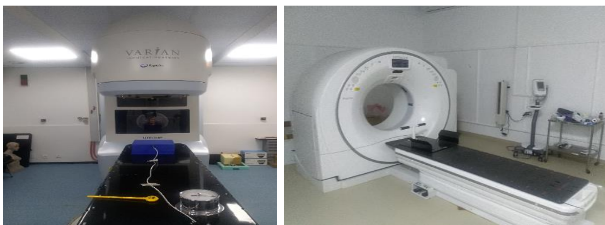
Figure 8: Installation of the LINAC and CT scanner.
