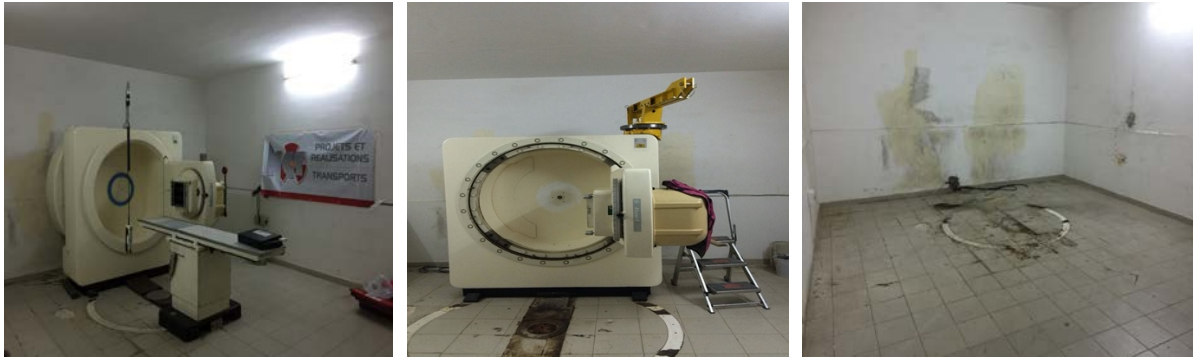
Figure 4: Cobalt decommissioning and removal
